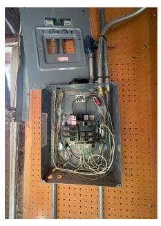
Branch Wiring Circuits, Breakers & Fuses: Wiring Method Romex, Concealed
